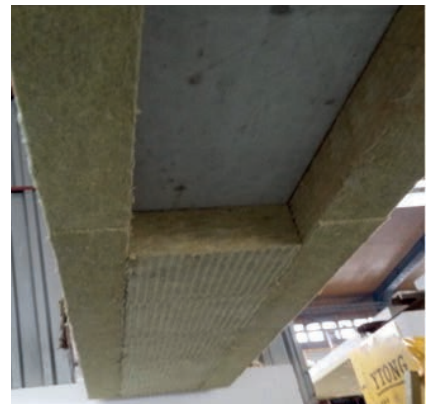
Fire protection on the bottom surface of the beam.
